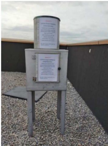
Figure 6. Rainwater Collector Device
